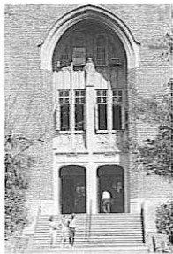
The Florida State University campus combines traditional gothic architecture with ultra-modern structures in a surrounding rich in trees and flowering plants. Large shade trees are unique to the Tallahassee area and make it one of the south's most beautiful cities.
