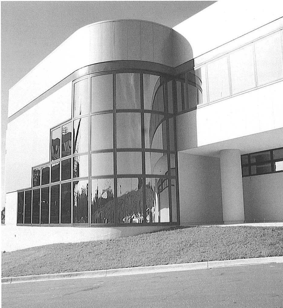
The ultra-modern Coyle E. Moore Athletic Center houses athletic administration, coach's offices, training facilities, locker rooms and the athletic dining hall. It's also home to the FSU Athletic Hall of Fame.
