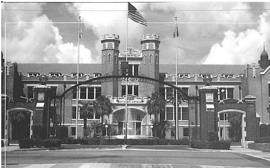
Westcott Hall was nearly lost when it was largely consumed by fire in 1969. The building was extensively rebuilt just in time to witness Florida State's rise to national prominence in the '70s and '80s.
