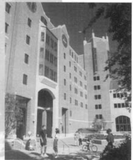
In fall 1994, the first tenants moved in to the east side of the $82 million University Center, a classroom-and-office facility at Doak Campbell Stadium. The stadium's south end zone also was enclosed and the adjacent Moore Athletic Center expanded. When the west side is completed in 1996, the University Center will provide 550,000 square feet of much needed academic space and a centralized location for student services.
