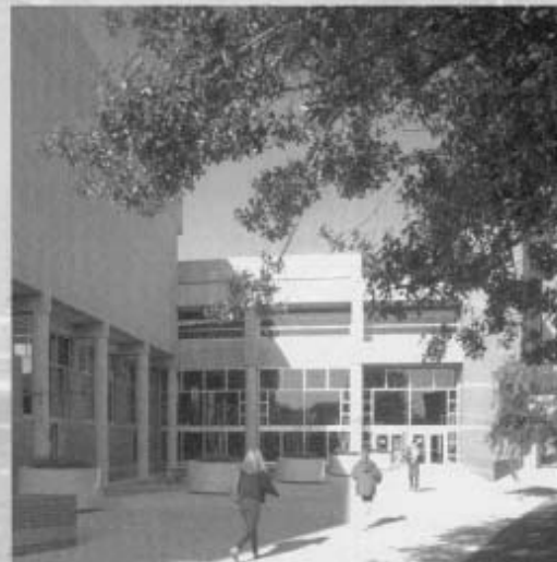
The Dr. Bobby E. Leach Center, a state-of-the-art student recreation facility, with an indoor pool, saunas, basketball and raquet-sport courts, was completed in 1991. And in June, a 2300 square foot free weight area was completed.
