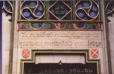
The façade at Dodd Hall
