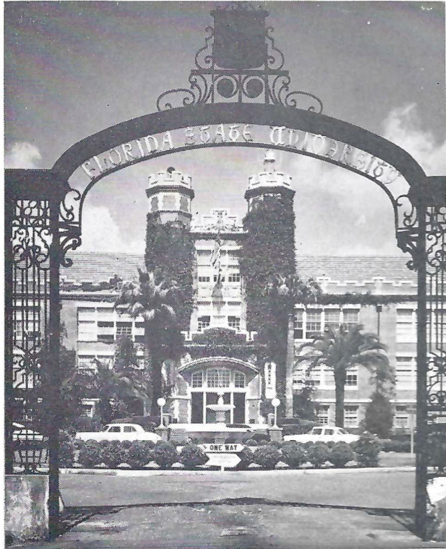
Main Gate, Administration Building
