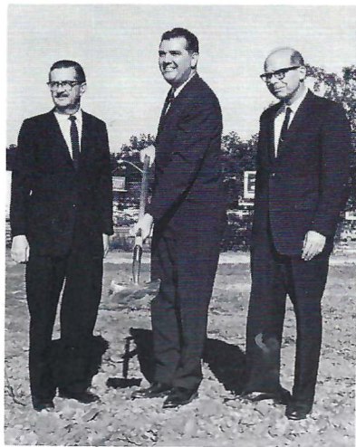
GROUNDBREAKING FOR FINE ARTS BUILDING —President John Champion, center, turned the shovel at the new Fine Arts site recently, assisted by Dr. Adolph Karl, left, representing the Department of Art; and Dr. Wayne Minnick, right, associate dean for the humanities in the College of Arts and Sciences and chairman of the Department of Speech.
