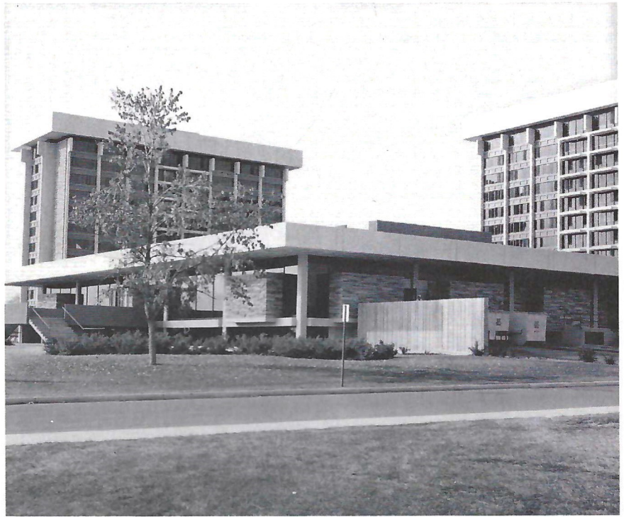
High-rise Dormitories Durward & Westphal Towers
